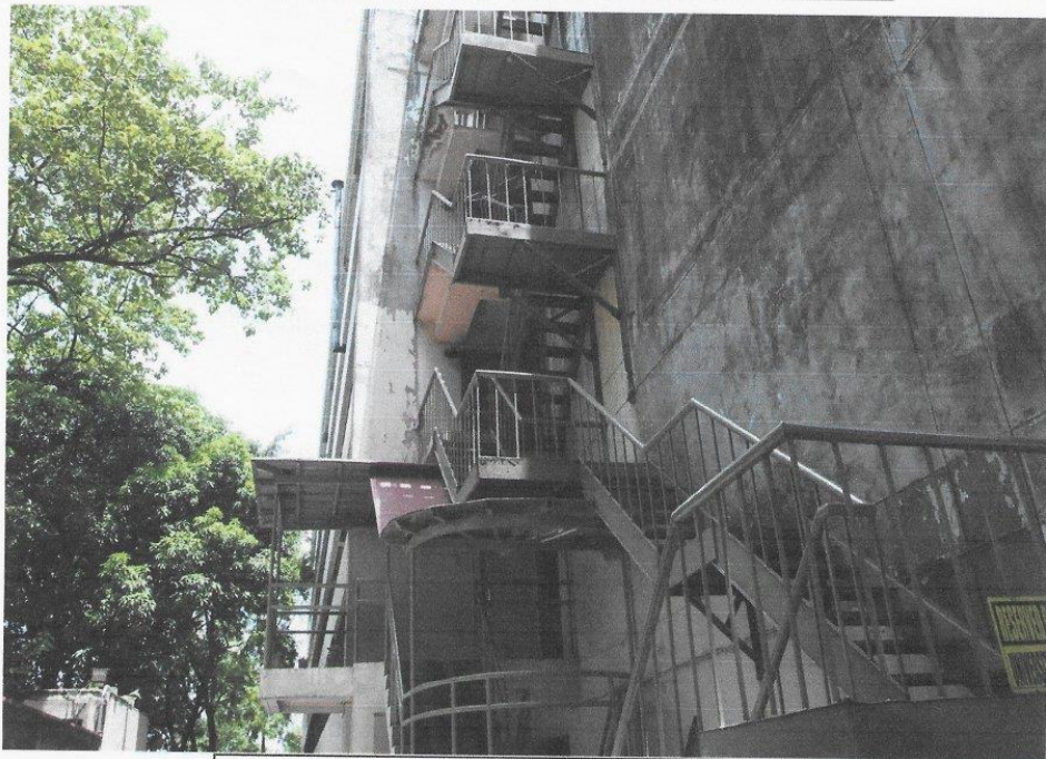
EMERGENCY EXIT AT MAIN BUILDING
